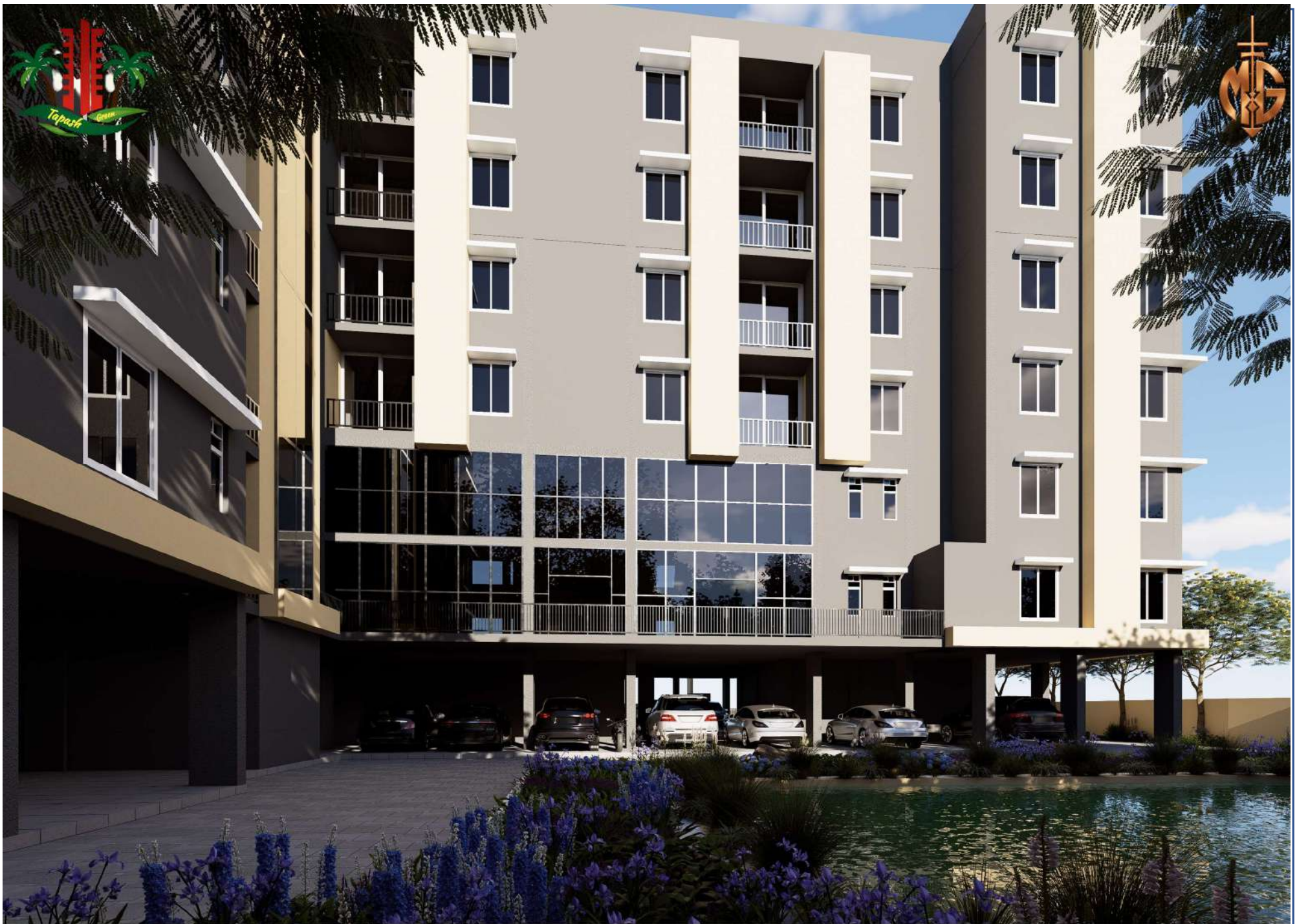
Elevation from the pond end
